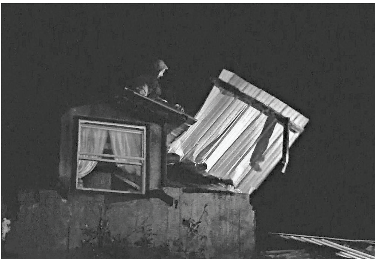
An emergency worker moves debris from a damaged house early Wednesday in Caddo Parish, La. A destructive storm is marched across the United States. KSLA VIA AP
